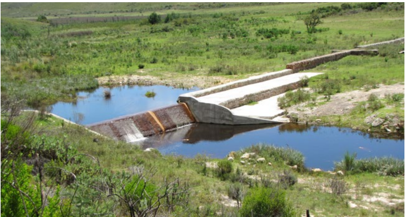
A concrete capped gabion weir on the Kromme River near Kareedouw. It was built by Working for Wetlands in the early 2000s under the supervision of the renowned wetland specialist, Japie Buckle. The weir was established to prevent headcut erosion of the palmiet-dominated wetland upstream. Photo: Japie Buckle
