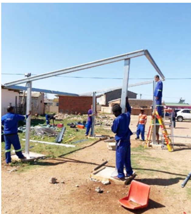
From left: Saltuba erection of PV Solar array. Saltuba Cooperative water capture system
